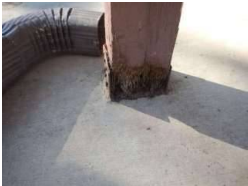
Photo 1-1 Multiple posts have rot at the base.
