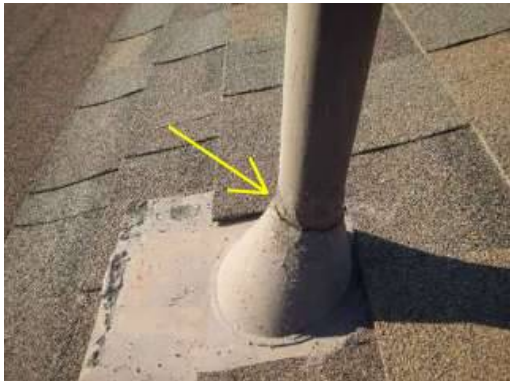
Photo 9-1 Recommend installing new flashing tape around the plumbing vents to prevent moisture from entering the structure.
