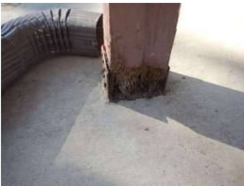
Photo 1-1 Multiple posts have rot at the base.
