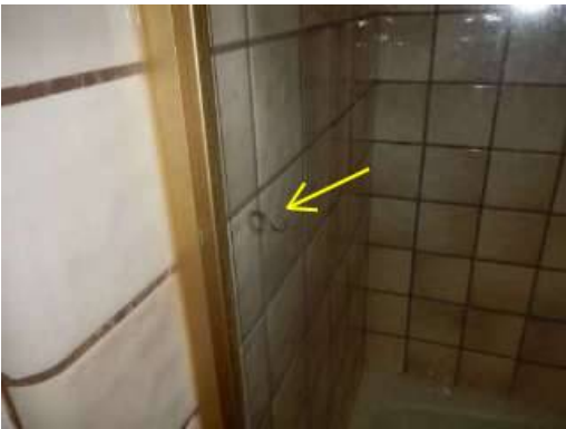
Photo 26-2 Missing handles to sliding doors.
