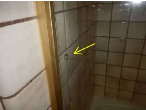
Photo 26-2 Missing handles to sliding doors.
