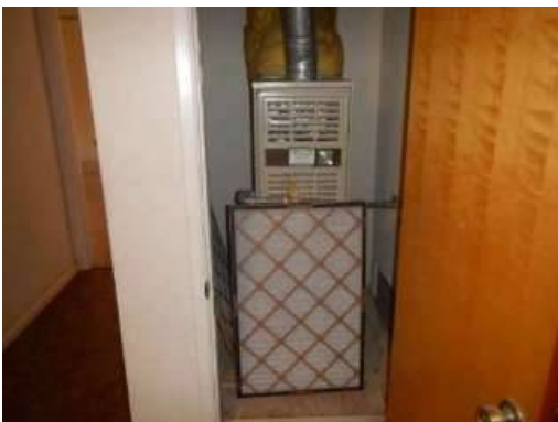
Photo 20-1 Unable to test this furnace do to the face that the gas valve was turned off. Recommend further inspection
